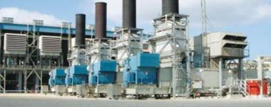
SGT-500 package in combined cycle configuration.
